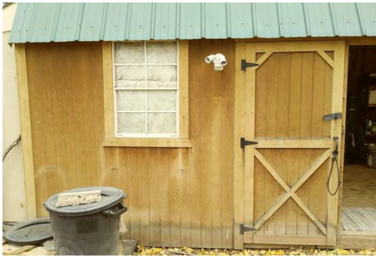
A shed converted to a walk-in cooler (photo: Patrick Jaramillo)
