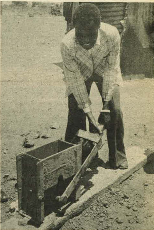
The NIEO fosters self-reliance and use of labor-intensive technologies. For example, the AFSC Zambian staff person, Alfred Kakoma (a construction trainer), in the picture above is using a simple hand-operated, soil-cement ram for making bricks from locally available materials. Building houses is part of the upgrading project being conducted outside Lusaka, Zambia, of which the AFSC is a cooperating member.
