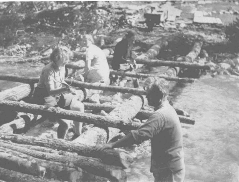
● Work campers helped the community people build a bridge across an unfordable stream at Shannondale, Missouri.
