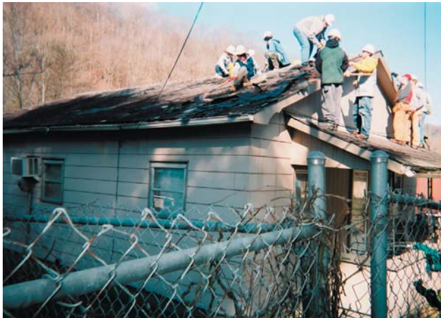
Home repair season is under way in Logan County, WV
